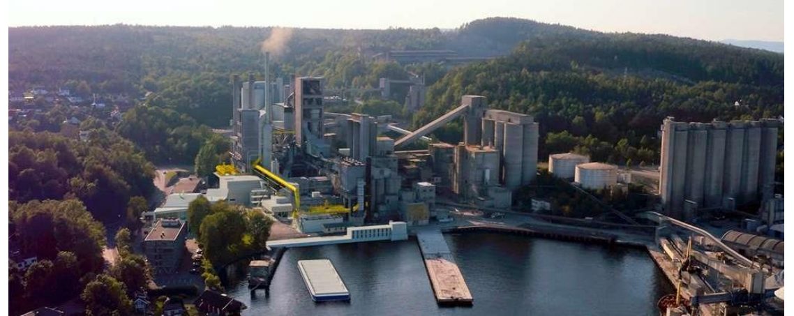
Norcem: Carbon Capture facility, CCUS (at HeidelbergCement, Norway)
