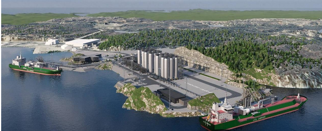
Photo: Northern Lights JV
