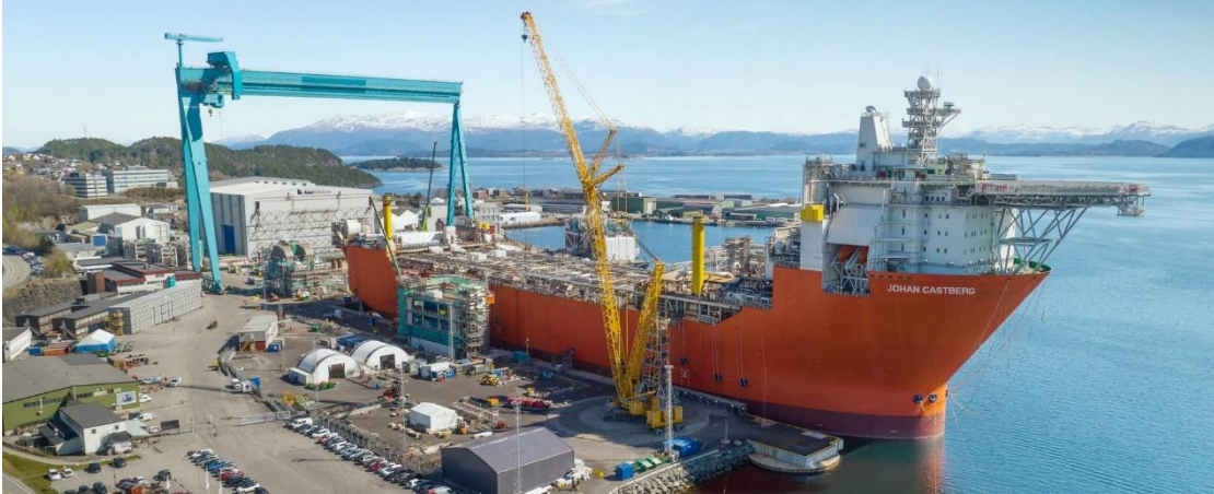
Johan Castberg: FPSO arrived, before topsides installed
