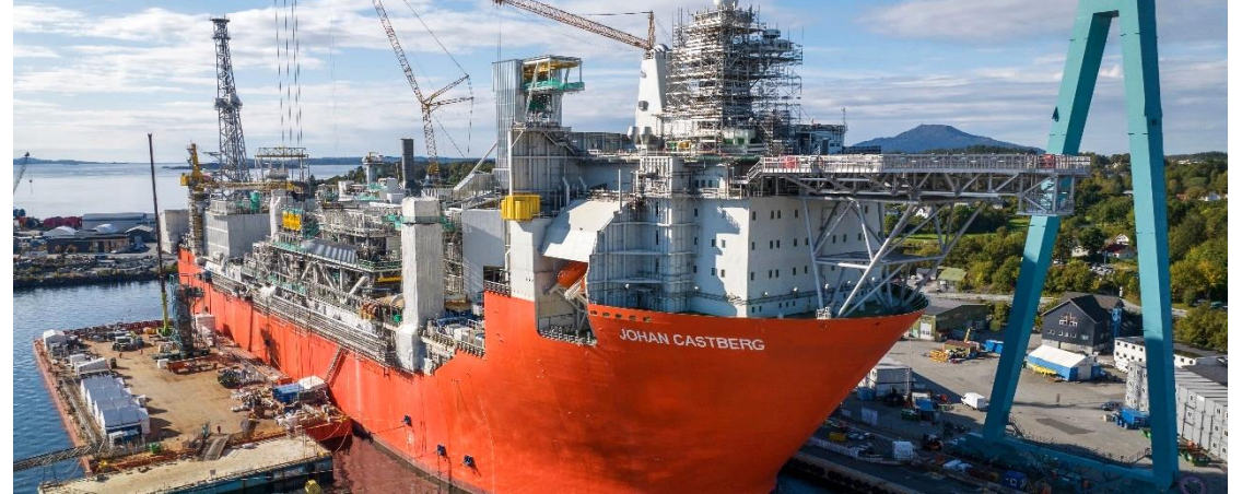
Johan Castberg: FPSO Topsides installed
